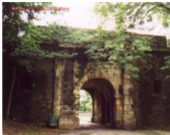
12. Gateway of Mirador Battery
