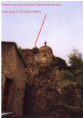
7. Storehouse behind Hornwork of Santa Clara and looking up to St. James Battery
