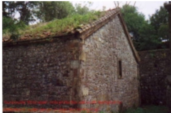
10. Gunpowder store again--note protective wall to south, but no protection to north, danger of Royal Navy blowing the store up.
