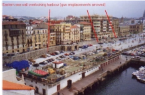
2. Eastern wall overlooking harbour (gun emplacements arrowed)
